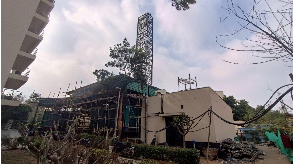
Photograph:- D.G Set with Acoustic enclosure and Adequate Stack Height
