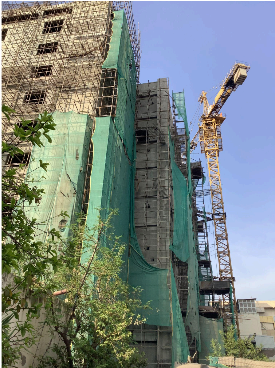
Photograph :- Construction Building
