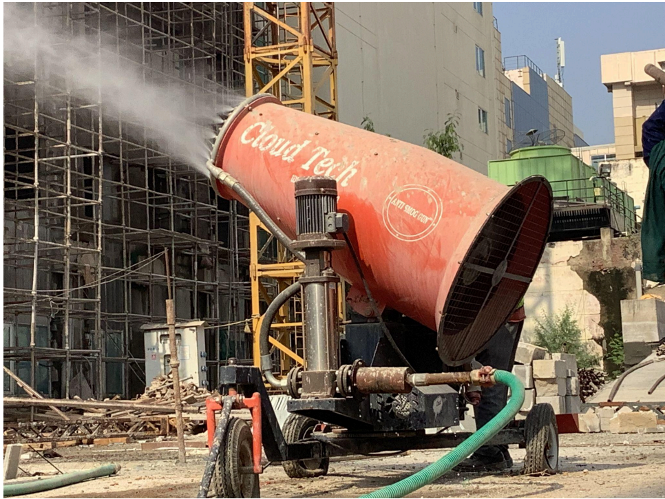
Photograph:- Anti-Smog Gun Installed at the Construction Site
