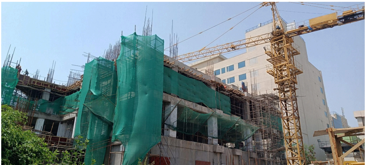
Photograph :- Under-Construction Building
