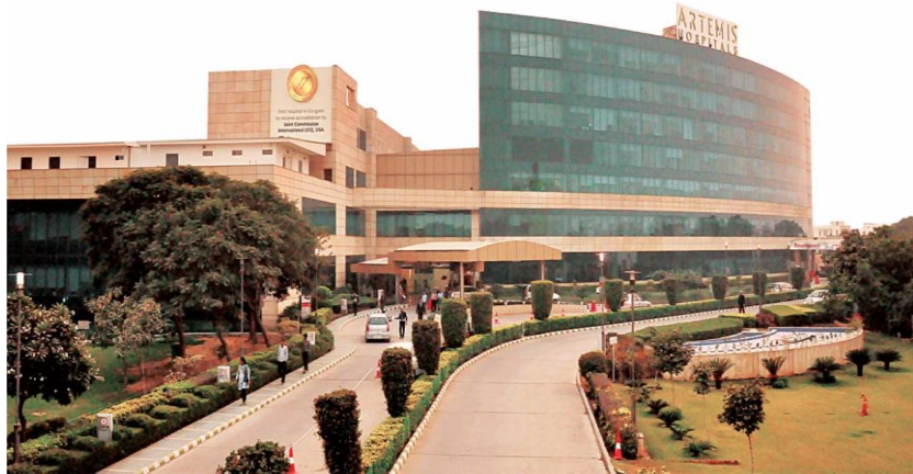
Artemis Hospital, Gurgaon
